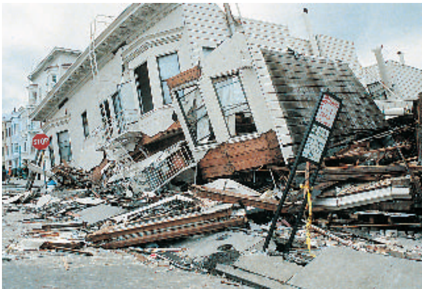
Figure 18 San Francisco's Marina district suffered extensive damage from liquefaction in the 1989 Loma Prieta earthquake because it is built on a landfilled marsh.
